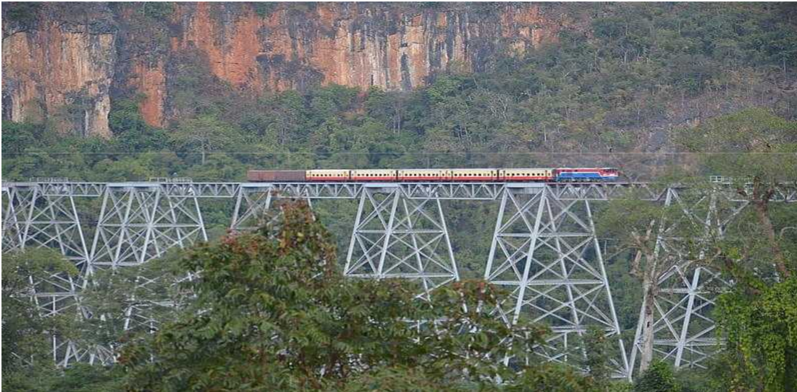
The Oldest Railway Bridge in Myanmar, "Gokteik Viadut" Construction start/end: 28-4-1899/1-1-1900 Total length: 689 Metres (2,260 ft)
